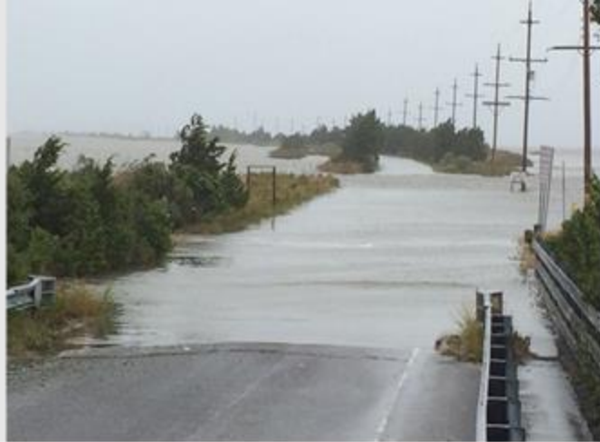
Figure 2: Great Bay Blvd., the road to the RUMFS, flooded during a nor'easter tidal event.
